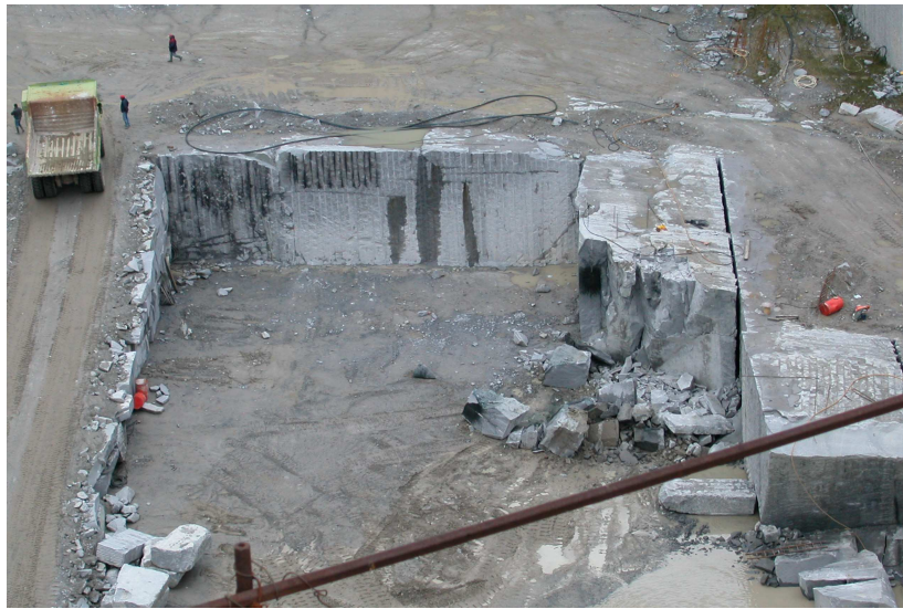
Figure 1: Granite quarry (MACEIRA). From the photo it is possible to observe the variety of difficulties arising from the extraction of a granite block
