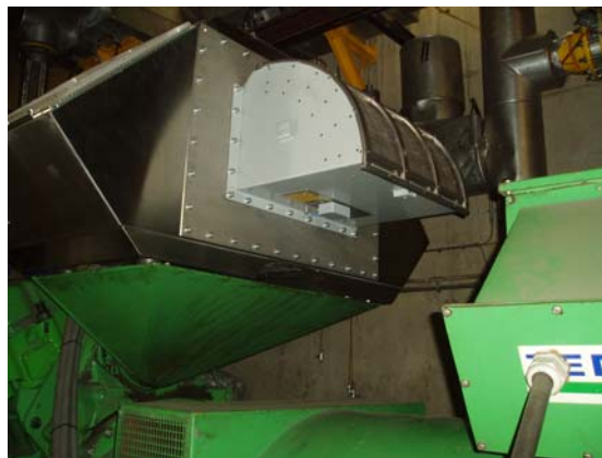
Fig. 3.44: Standard air filter housing (left); Pressure relief device mounted on air filter housing on the Güssing gas engine (right)
