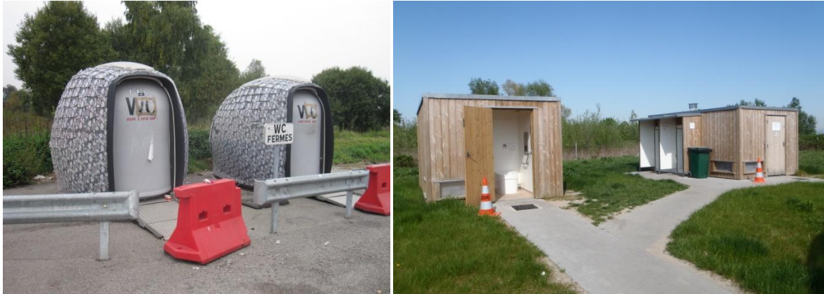
Landgraben rest area: Flushing toilet (left) before Sanimassive (right)
