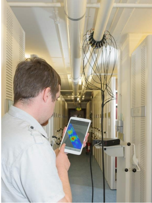
Figure 7. SprinkTest integrated system.
