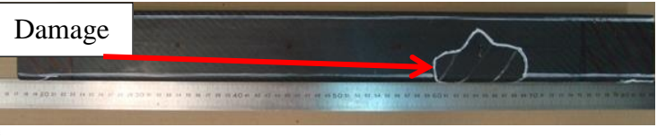
Figure 6: US inspection of beam No. 4
