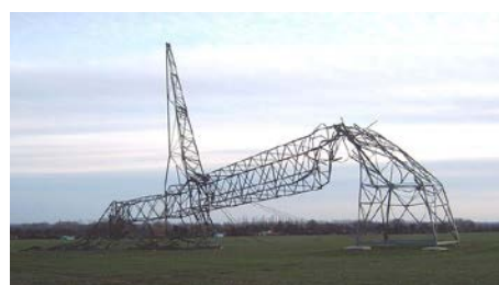
Figure 2.2 Damaged power pylon due to high winds
