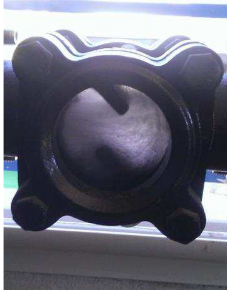
Figure 20. View of the steam generated with solar-only mode, after the collector outlet.
