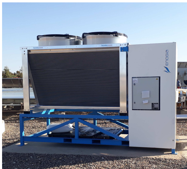
Figure 12. View of ORC power unit coupled to the air cooler.
