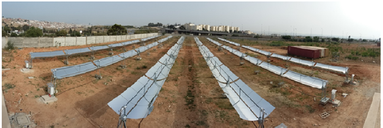
Figure 15. View of the P3 solar field after collector installation.
