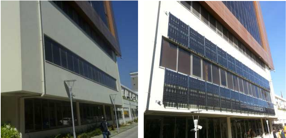
Figure 4. View of prototype façade (Southeast): before and after installation of the PV modules.
