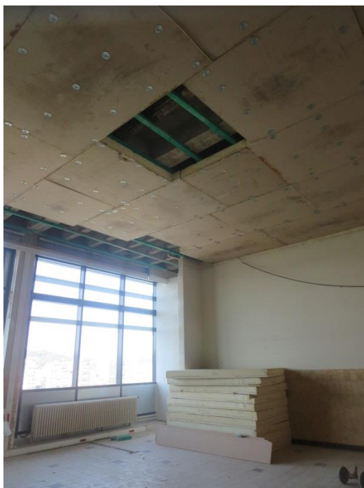
Figure 5.6: PIR foam panels with embedded PCM installation works in Liège.
