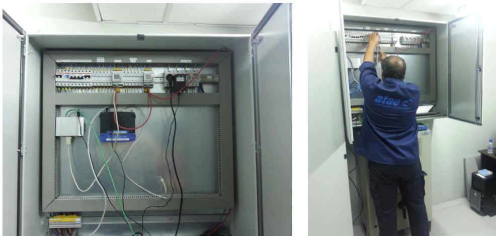
Figure 5.3: Bricker Cabinet installation in GEX building
