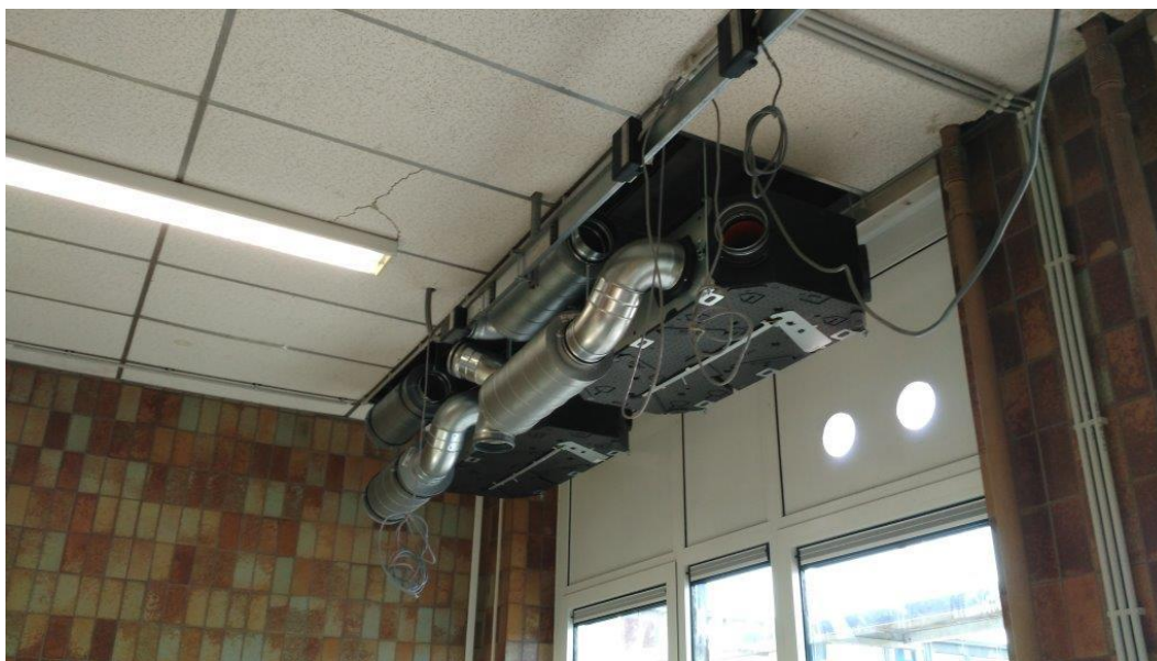
Figure 5.5: GREECOM first double flow unit installed at MONTH 36.
