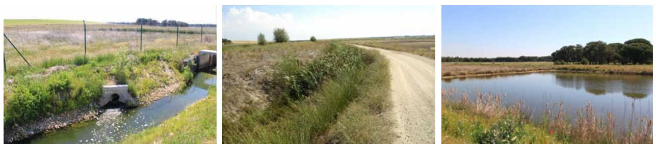
Fig. 7: 'Triplet' in the Santiuste basin to study water quality improvements for treated wastewater. Inflow of treated wastewater into the canal system (left), section with dense plant growth as a 'green biofilter' (middle), and constructed wetland (right).
