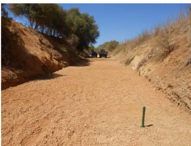
Fig. 4: Prepared river bed at the Rio Seco to allow efficient infiltration of water (left), and response of groundwater levels below the river bed during a strong rain event in January 2016 (right).
