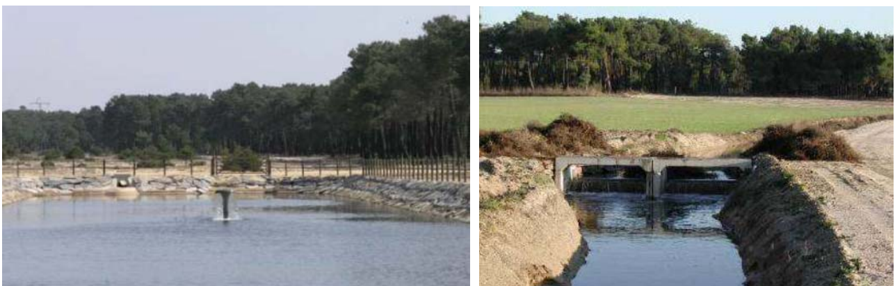
Fig. 6: Typical infiltration pond during a wetting phase (left) and typical channel for the diversion of water for MAR infiltration (right) in the Arenales region.
