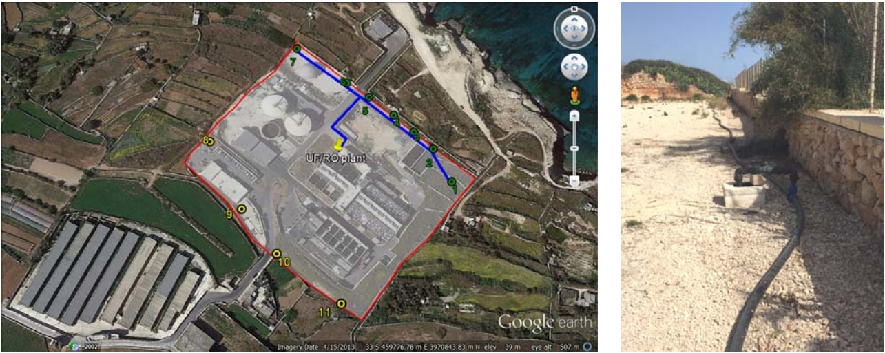
Fig. 16: Location of the Malta South wastewater treatment plant and implemented infiltration wells for the polished effluent (green) and up-gradient monitoring wells (yellow) for control of groundwater levels (left). Detail of the distribution network and infiltration gallery (right).
