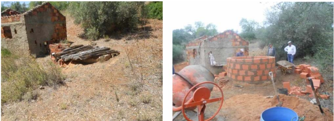
Fig. 5: Old large-scale diameter well before (left) and after rehabilitation (right).
