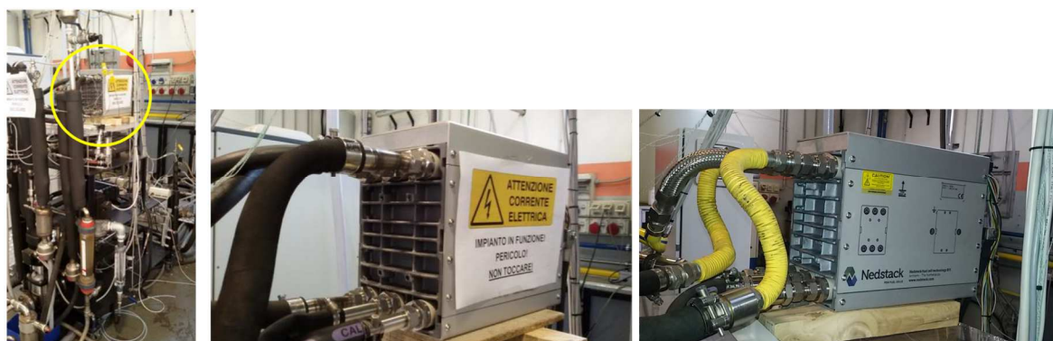
Figure 2: Nedstack FC stack S0335 – 40 cells
