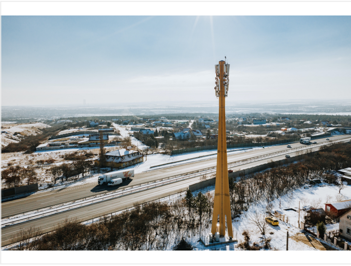
Ecopol wooden structured telecom tower
